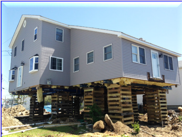
Home elevation after Superstorm Sandy in New Jersey
